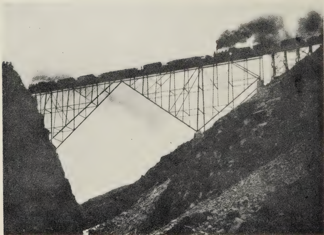
Steel bridge near White Pass.
